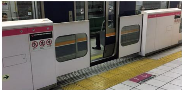
The position of conventional platform screen doors is fixed.
